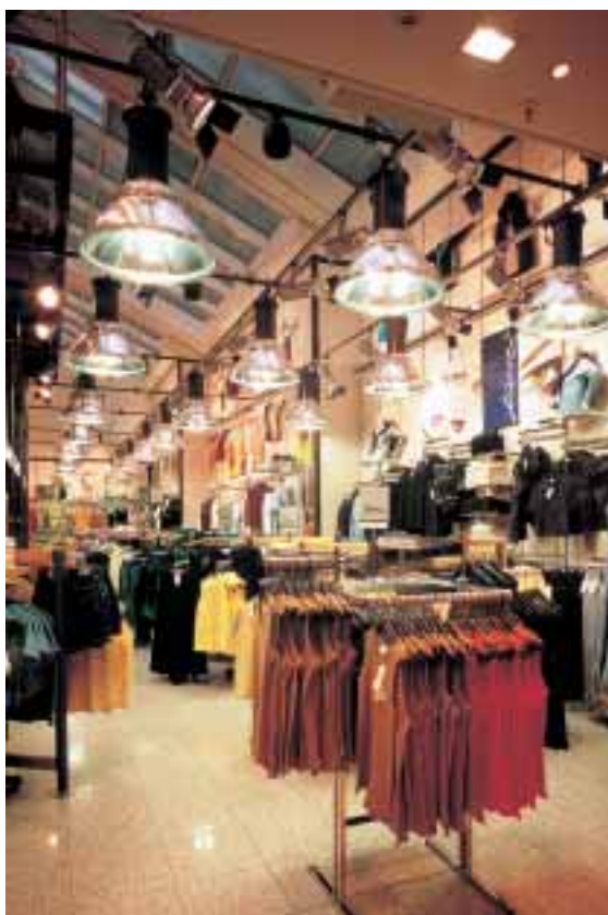
An interesting example of OSRAM DULUX® F lamps in vertical downlights.
