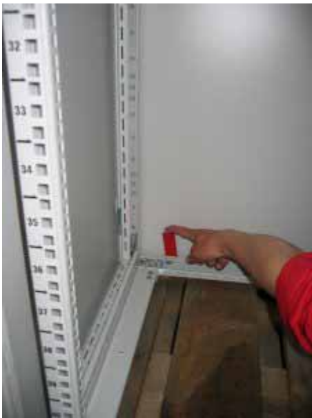
8. Side- and back panel are secured by a red lock at the bottom.
