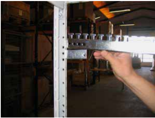
4. Cableguide is placed in the back of the panel.
